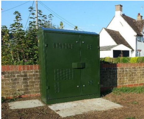
Superfast Broadband Street Cabinet at junction of Joyces Road and Van Diemans
